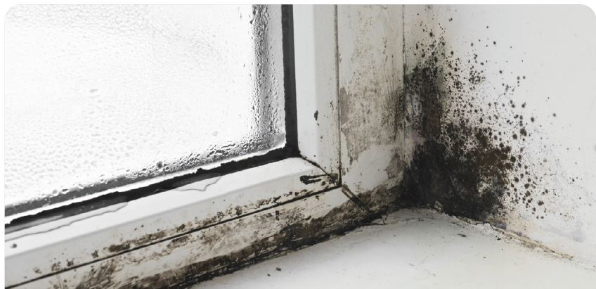
Example of black mould forming around a window frame
