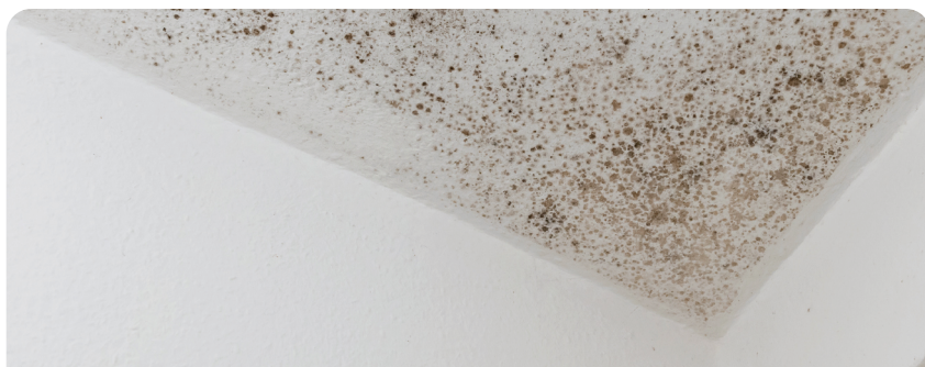
Example of mould caused by loft insulation cold spots
